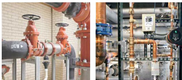
Pictured Left: Watts Backflow preventers & Pictured Right: The Powers IntelliStation® I (Credit: Watts Water Technologies)
